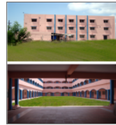
Back side of the entire building(s)/block
